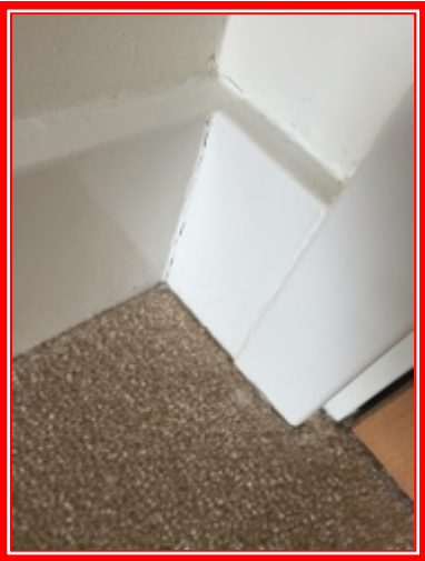
7.5.1 Skirting has a few marks and cracking.
