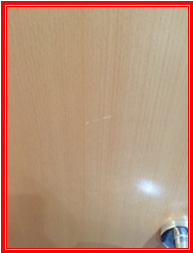
3.3.1 Door has a few marks, and creeks/squeaks when opening/closing.
