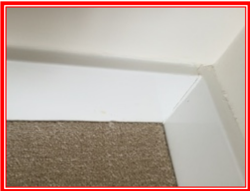
5.5.1 Skirting has hairline cracking.
