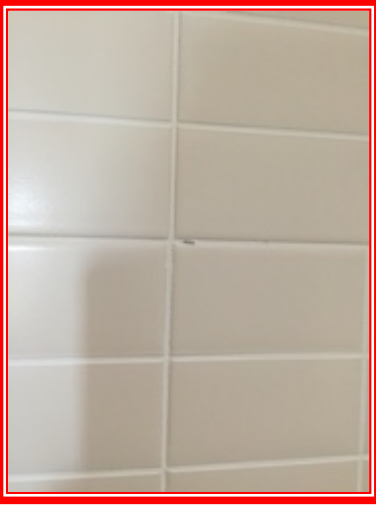
6.5.2 Grouting has a mark.
