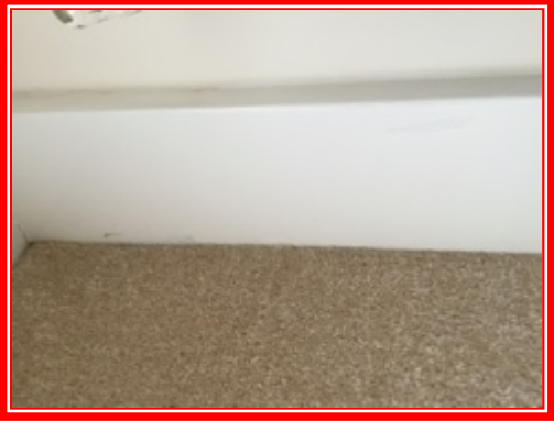
7.5.1 Skirting has a few marks and cracking.
