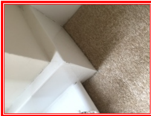
5.5.1 Skirting has hairline cracking.
